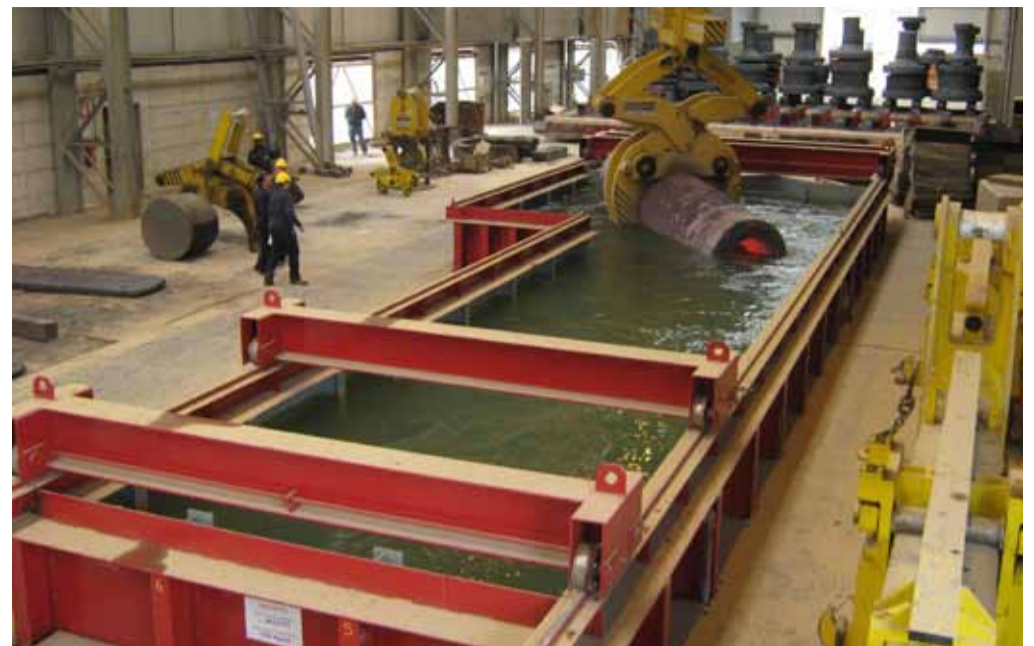
New water quenching tank at FOMAS
