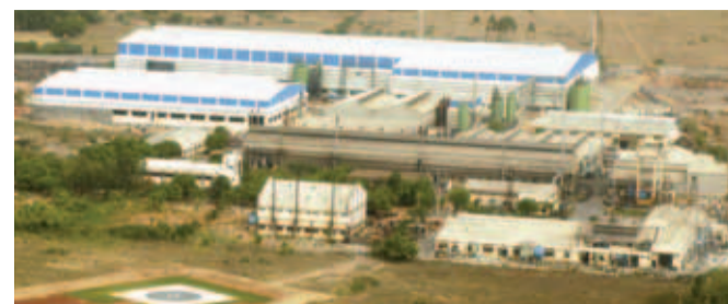
View of the Sanmar Foundry Steel Foundry complex consisting of a sand foundry with a capacity of 25,000 MT per annum, an investment foundry with a capacity of 1200 MT per annum and a well equipped CNC machine shop.
